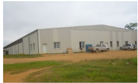
Figure 1: The raceway of HYDROFISH in the village of Anna to 9 km of Binger Ville. Source : [3]
